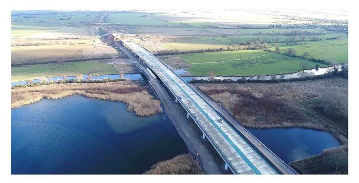
**Section 3:** Surfacing on the Huntingdon southern bypass has resumed, transforming long stretches into recognisable road. Less obvious, but essential, is the mainline drainage work, which is progressing well, with completion expected in the spring. Work to create the embankments for the new bridge at New Barns Lane is nearly complete and the beams for the bridge are expected to be installed in April.
